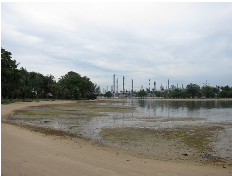
Fig. 6: The SHELL oil refinery can be seen from the background of this image of Pulau Hantu Besar (Ng, 2011)
